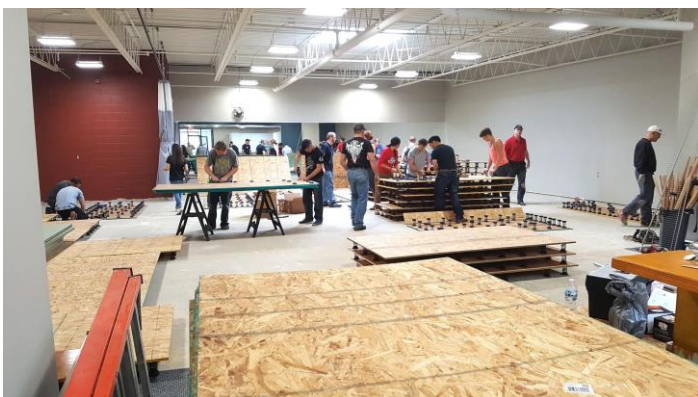
Suino Sensei's students helping construct a special sprung floor for the mats in their new dojo
